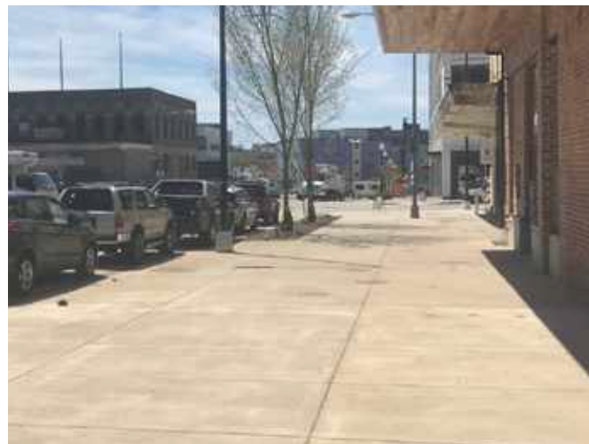
CONCRETE GROUND PLANE
